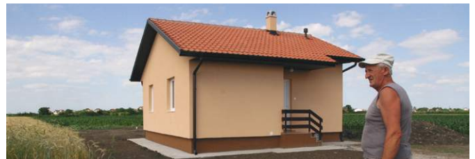
Temerin, Serbia Construction of over 300 pre-fabricated houses throughout Serbia
