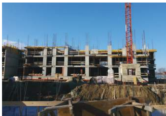
Construction of 235 apartments in Ovca, Belgrade
