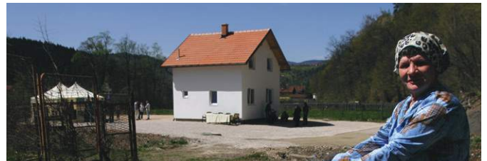
Olovo, Bosnia and Herzegovina Provision of building material packages to 20 families throughout BiH
