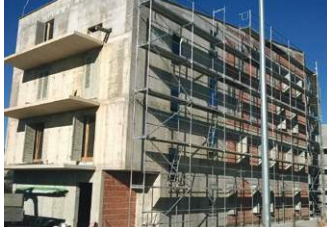
Construction of 40 apartments Knin, Croatia
