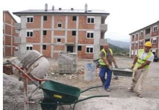
Construction of 120 apartments Konik Camp, Montenegro
