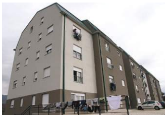
Construction of 62 apartments Niksic, Montenegro
